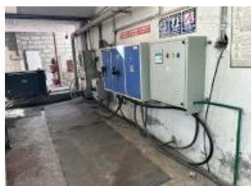
36. Anti-shock rubber mat provided beneath electrical panel.JPG
