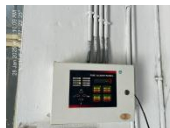
29. Fire alarm control panel.JPG
