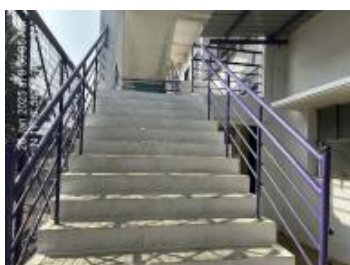
34. Hand Rail provided on both ends.JPG
